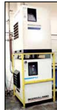
Ingersoll Rand Tm300T Refrigerated Air Dryer
