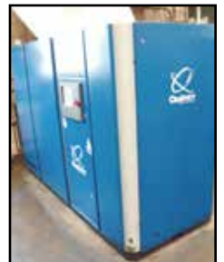
Quincy Mdl. QGV-60 Rotary Screw Type Air Compressor
